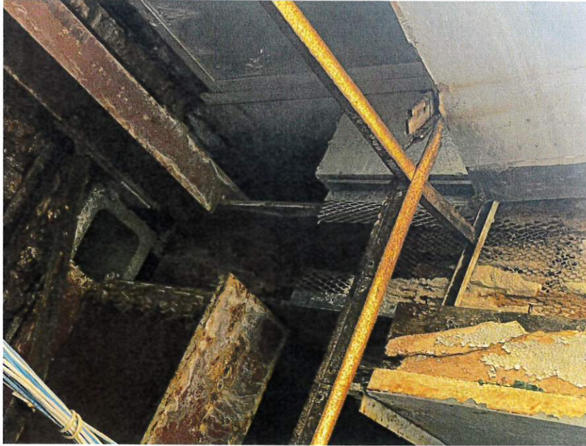
9. Floor Beam at Column Between Windows
