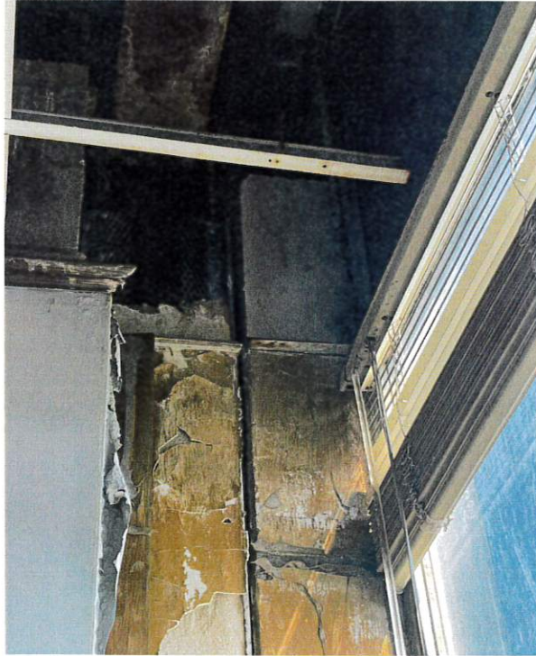
3. Precast at Column
